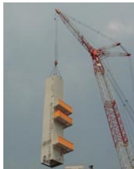
Fig. 2 Installation of divided cold box.
