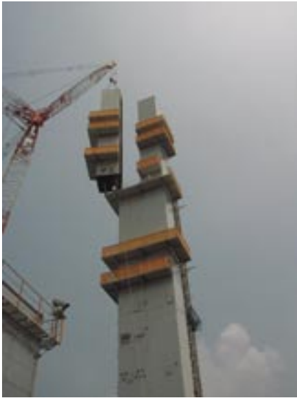
Fig. 3 Installation of cold box.
