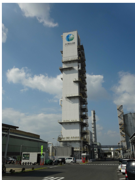
Figure 2 Oxygen-18 separation unit (No.3)
