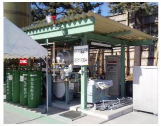
CO<sub>2</sub> liquefaction system
